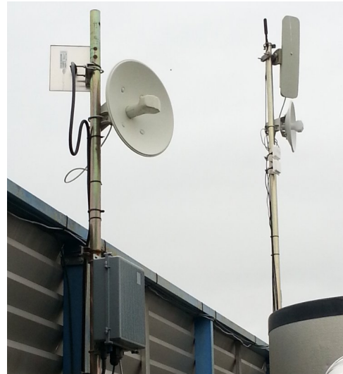
Figure 2. Super node with outdoor hardware for wireless links between community nodes
